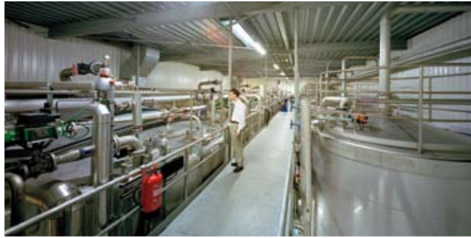
Proces installation Nedalco
