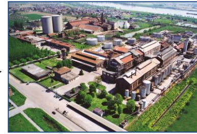
ADRIA (RO) Fermentation Plant as industrial pilot 1600 m3 fermentation capacity /Mater-Biotech
