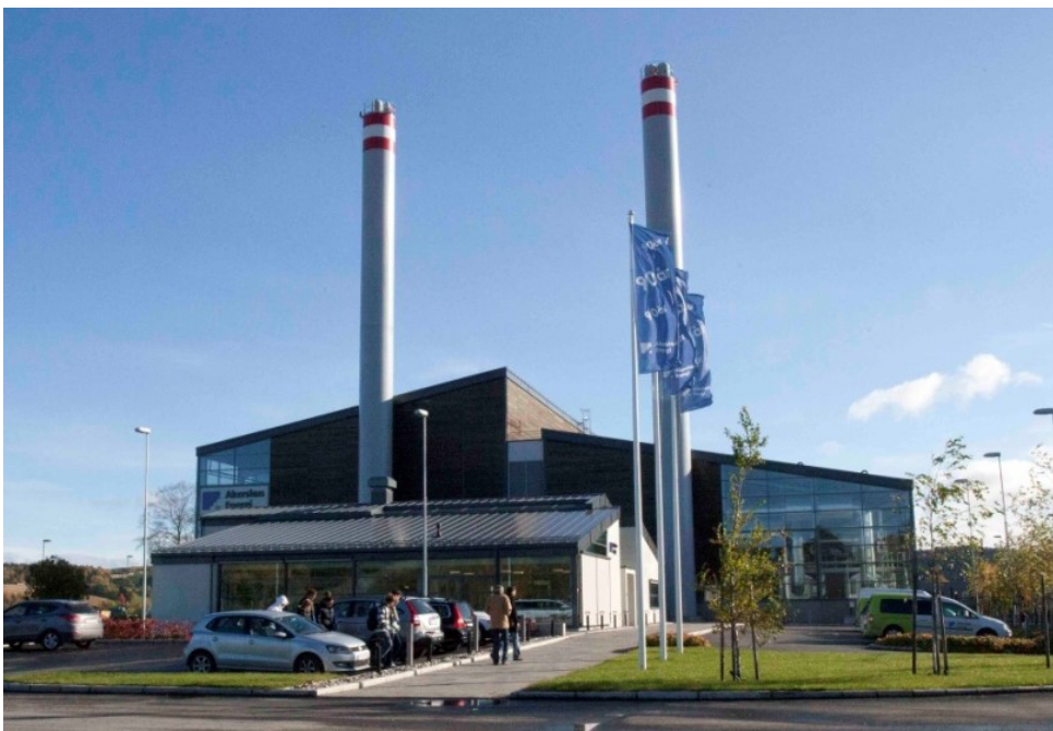
Figure 14.10. Akershus energy park in Norway.
