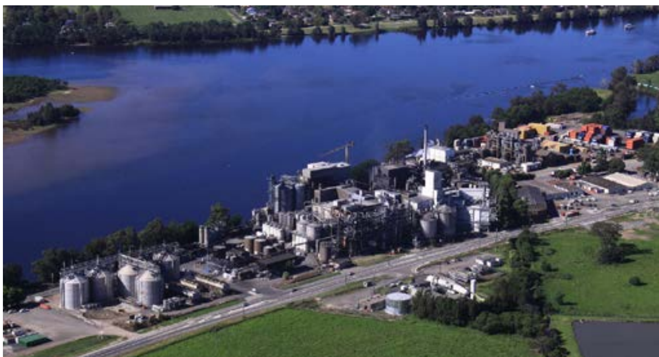
Figure 14. Bomaderry Plant, New South Wales, Australia (Dec 2011) [Manildra Group]
