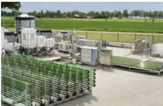
Figure 31. AlgaePARC Pilot Facility [Wageningen UR]
